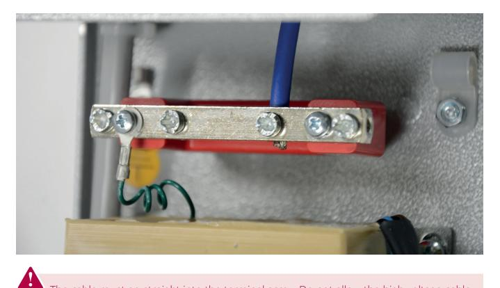
The cable must go straight into the terminal screw Do not allow the high voltage cable to loop or crisscross.
