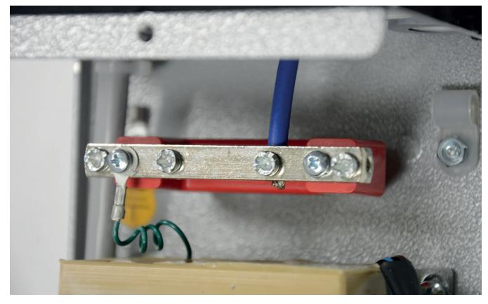
11. Loosen one screw on the terminal block and connect cable wire. Tighten screw.
